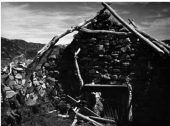
In parts of the Hebrides, another solution evolved, with the inner edge of thick, load-bearing walls carrying short timbers (often driftwood) which met at the roof
