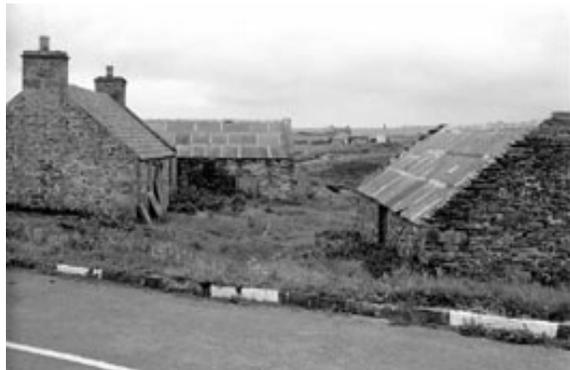
A few areas, notably Caithness and Orkney, were lucky enough to have hard flagstone rock, which could be split into thin sheets without their cracking. Here (previous page, right) at **Park**, on the island of **Hoy, Orkney**, the size of these slabs is clearly apparent.
