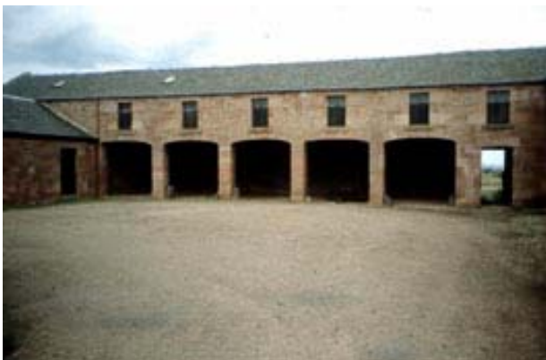
This fine granary at Thurston Home Farm, East Lothian , is sited (as usual) above cart bays.
