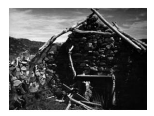
birch, were available, they were lashed together so that several sections formed one arch. This **ruined house** at **Gairloch, Rossshire**, has crucks made from two timbers pegged together.
